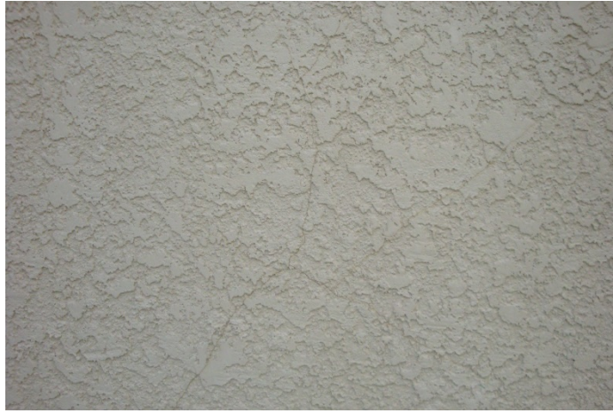
Hydration Cracks
