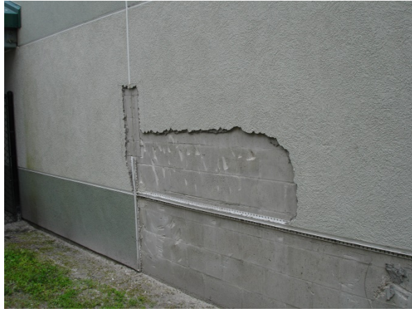
Deer Park School Stucco Repair
