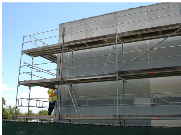
Oak Park School - More Stucco Repairs
