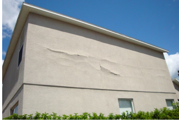
Stucco Delamination
