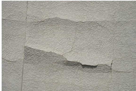
Serious Cracking
