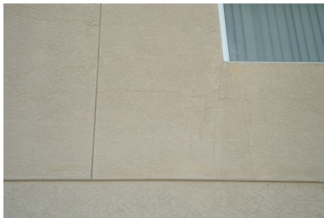
Hydration Cracking
